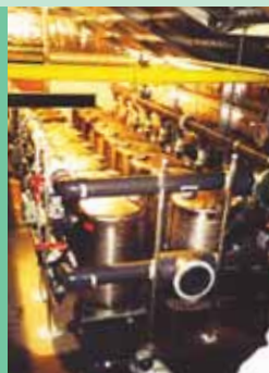
Pre snow gun water polishing at ski resort in Australia. Water supply from local storage dam.
